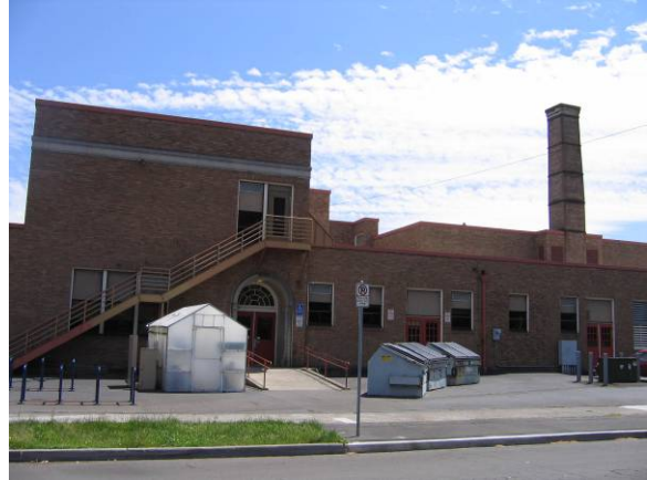
West elevation facing southeast
