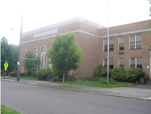
East elevation facing northwest
