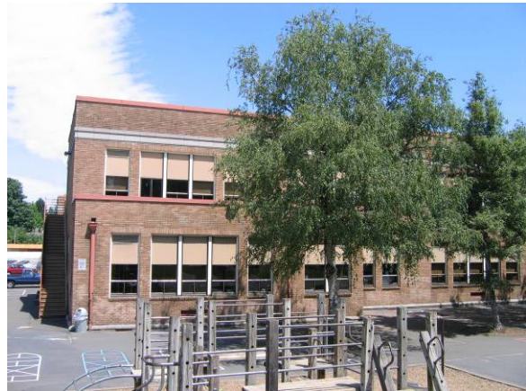
South elevation facing northwest
