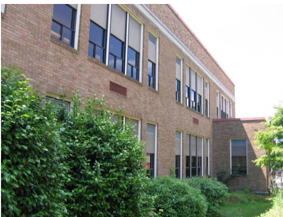
North elevation facing southwest
