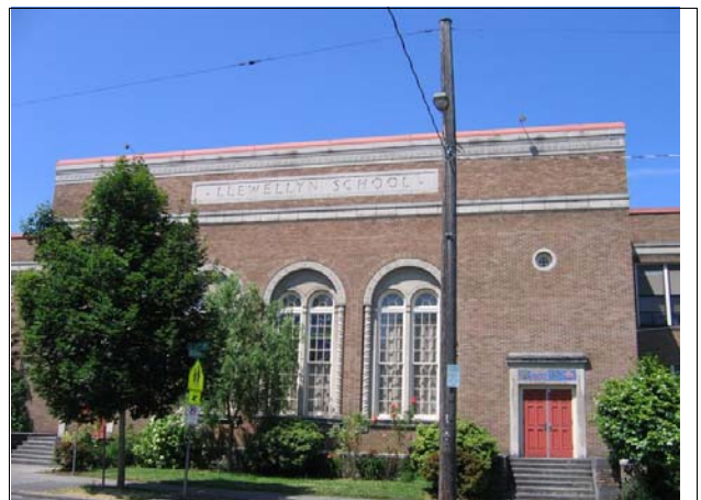
East elevation facing west
