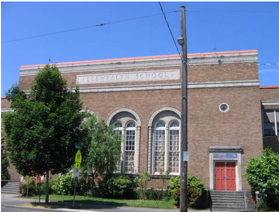
East elevation facing west
